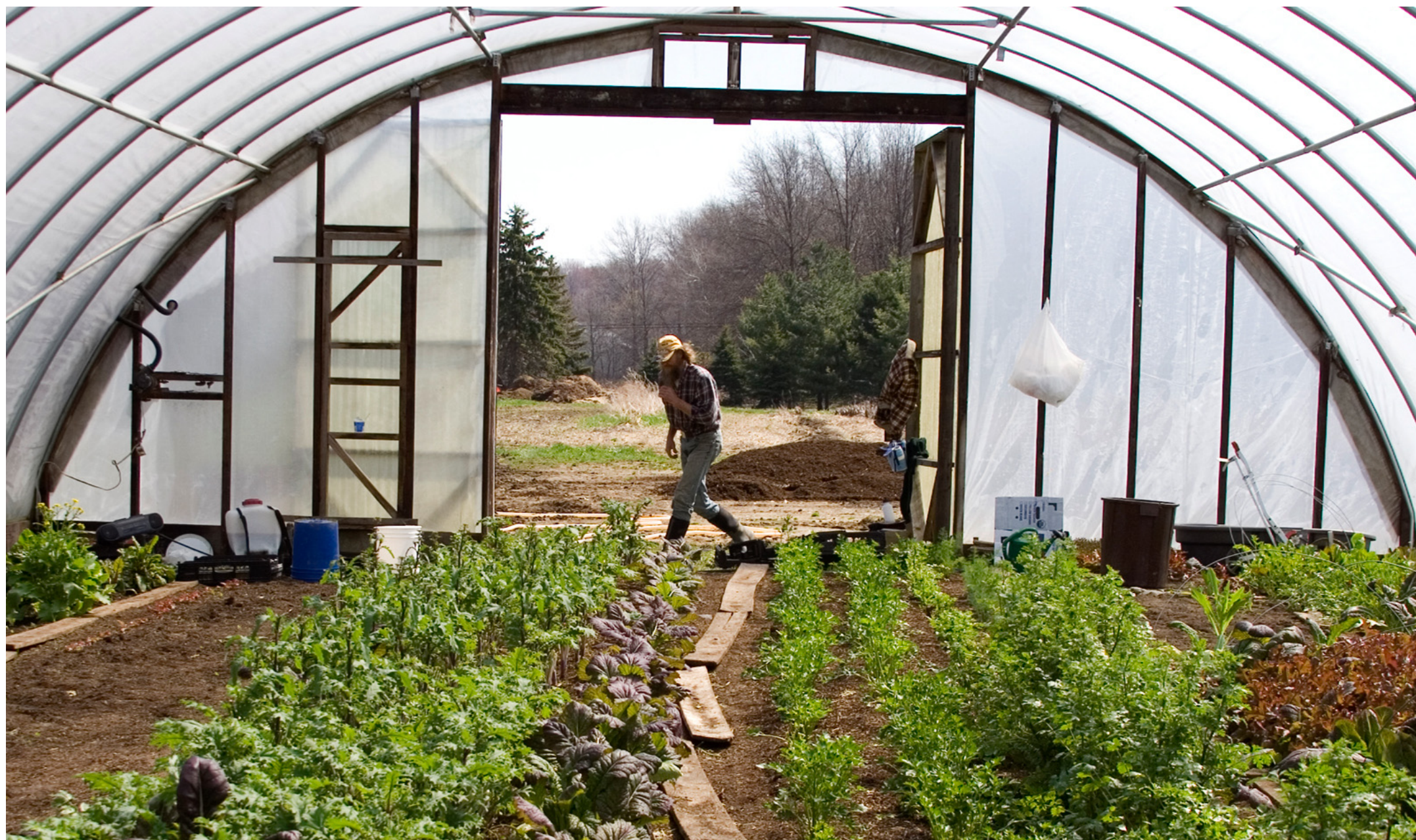
Bill earns his income in the winter by growing crops in a hoop house that he built himself. The plastic between the metal bars fills with blowing air from an inserted tube and acts as insulation to keep out the cold winter air.
